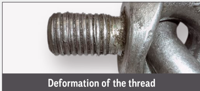
Deformation of the threaded bolt
